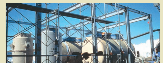
Wastewater treatment building (Photo taken during construction)
