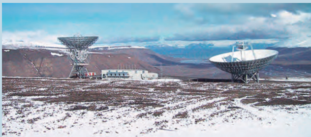
EISCAT Svalbard radar
